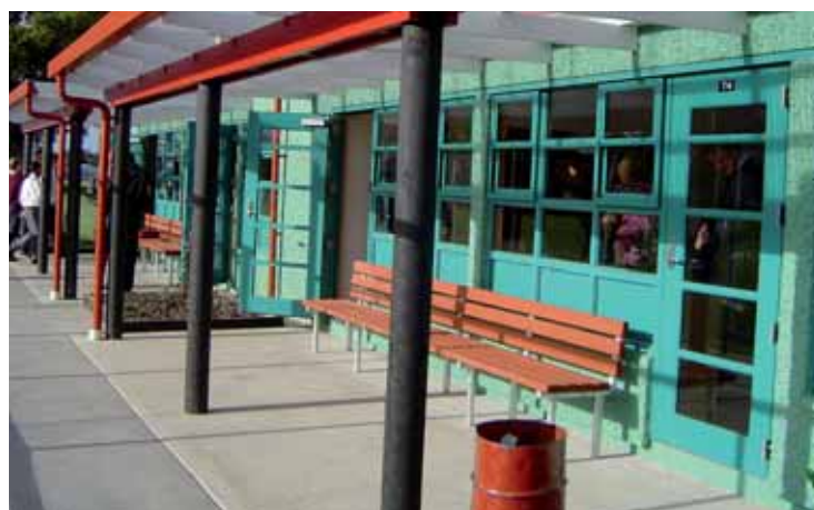
The exterior of St John's College, Hastings new Technology Suite
