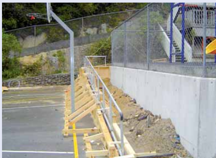
Access ramps under construction at St Benedict's, Khandallah
