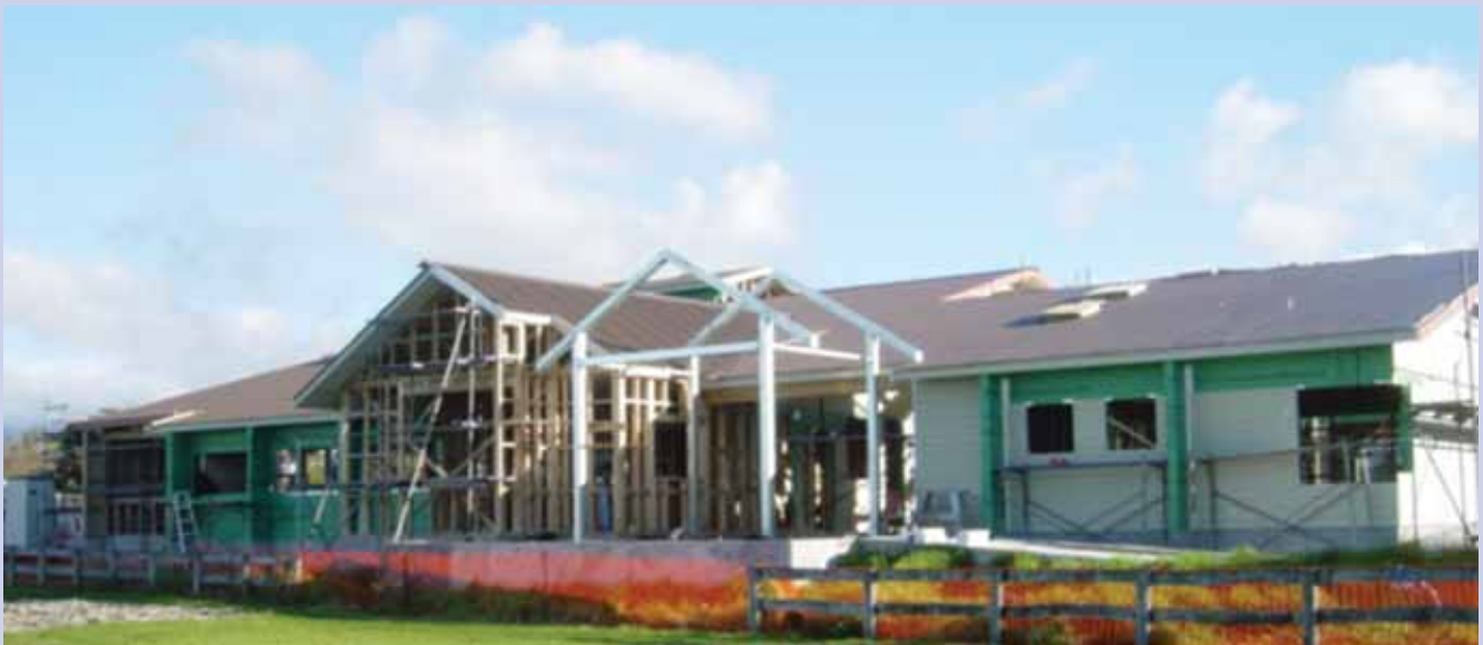
Francis Douglas Memorial College Technology block in progress
